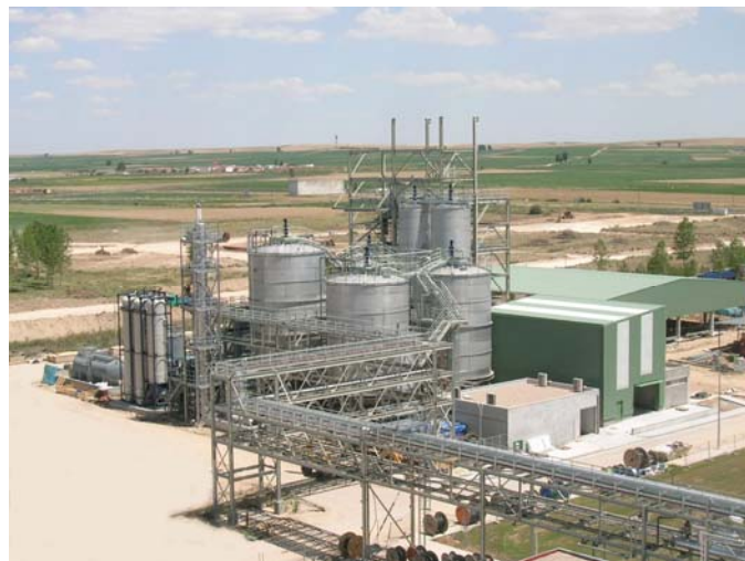
Grencell's bioethanol pilot-plant under construction at Babilafuente (Salamanca, Spain)
